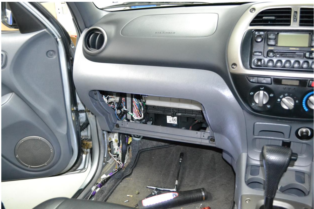
4) Side trim now removed
